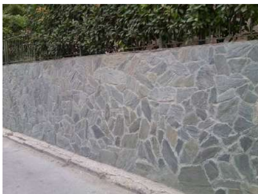
Figure 10. Green schist facade cladding [URBANTEK-Radovis]
