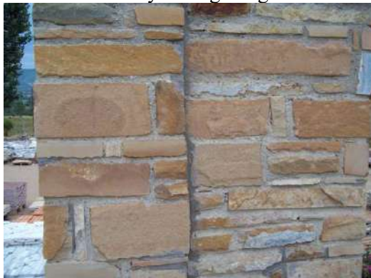
Figure 16. Usage of sand stones as architectural-construction stone material [URBANTEK-Radovis]
