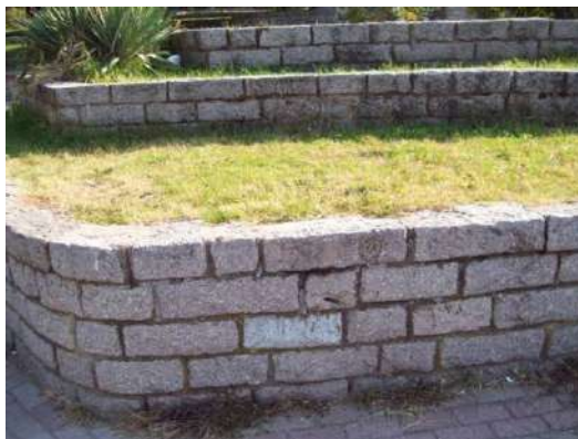
Figure 4. Andesitic wall construction - Public School "Vanco Prke" in Štip [Lj.Kulakov 2011]
