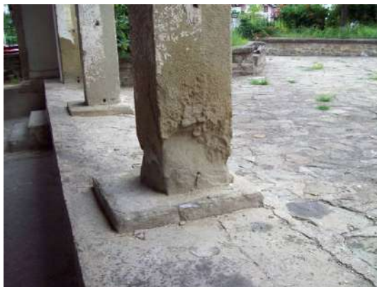
Figure 17. Destructive capillary moisture to sand stones at Sv.Nikola church in Stip [Lj.Kulakov]
