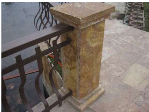
Figure 12. Vertical and horizontal travertine lining [City Park - Skopje]
