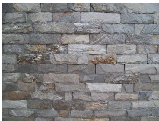
Figure 11. Green schist facade cladding [URBANTEK-Radovis]
