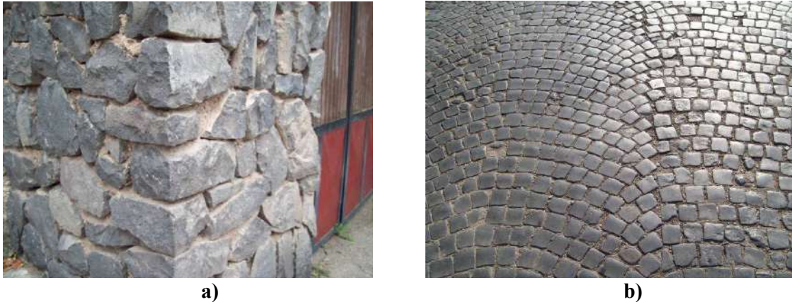
Figure 3. Basalt a) Wall b) Macadam road construction - Stip [Lj.Kulakov 2011]
