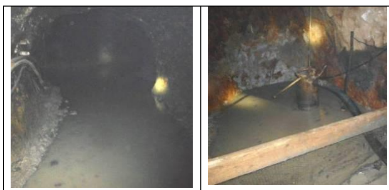
Figure 1. Temporary water halls with portable electric pumps
